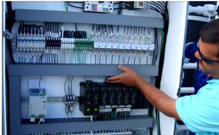
(Above) Mike Newell describes the interior workings and wiring of the field- located Programmable Logic Controllers (PLC), and circuitry of the Polaris Hands on Trainer.
