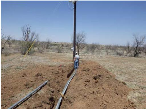
*(Top left)* Conduit installed to the Big Country Electric Utility pole – for power to the ‘core’ of the field lab.
