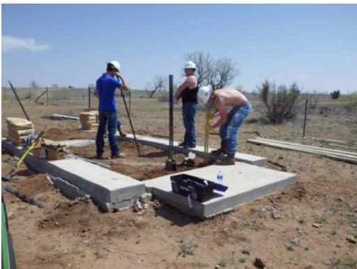
*(Bottom left)* In the Field lab, anchors holes were dug by students Kyler Free, Kylon Davis, and Tyler Hammond and Anchors set to anchor the Control Room to the ground (wind speeds can exceed tropical storm wind speed).
