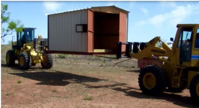
*(Top left)* The 14 foot X 9 foot (interior) control room was awkward to move requiring two large pieces of equipment to lift it off a trailer in a delicate balancing act.
