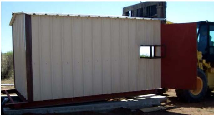
*(Bottom left)* Only one large fork lift was needed to maneuver the control room to its resting place atop the foundation slab.
