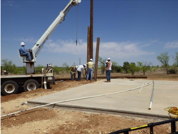
*(Left)* Lineman class setting pole 3, of the interior lab power transformer mount poles, next to the concrete slab for the Polaris H.O.T.
