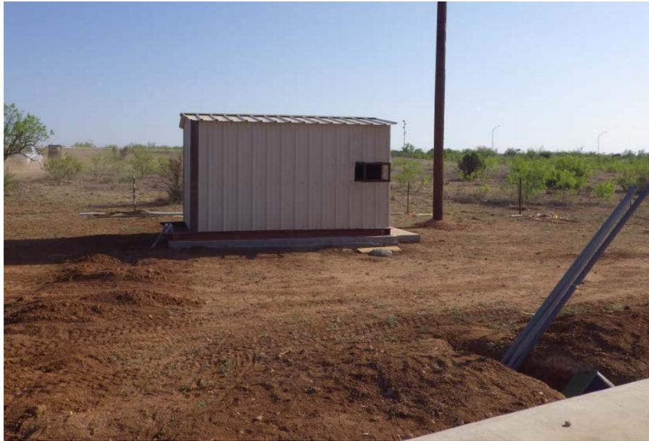
*(Above)* Control Room set on slab, after the control room was set in place, the lineman class installed the pole. Pole set for wireless antenna (to provide internet connectivity for field activities).
