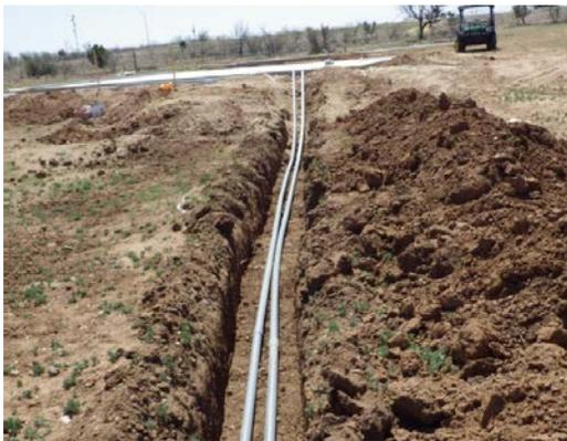
*(Middle left)* Power Conduit to the center of the field lab. Prior to setting of interior poles. Two lines run, one for future use.
