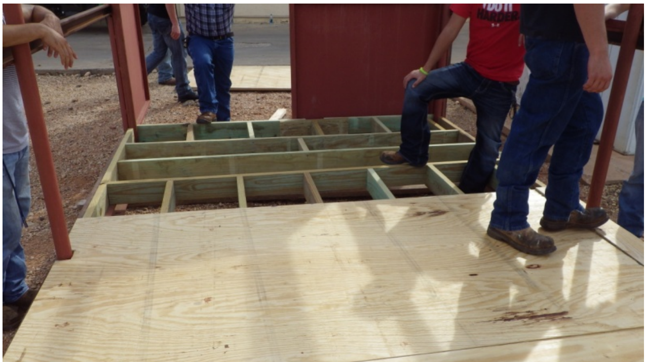
(Above) Progress continues to be made on the control room, with the addition of a floor.
