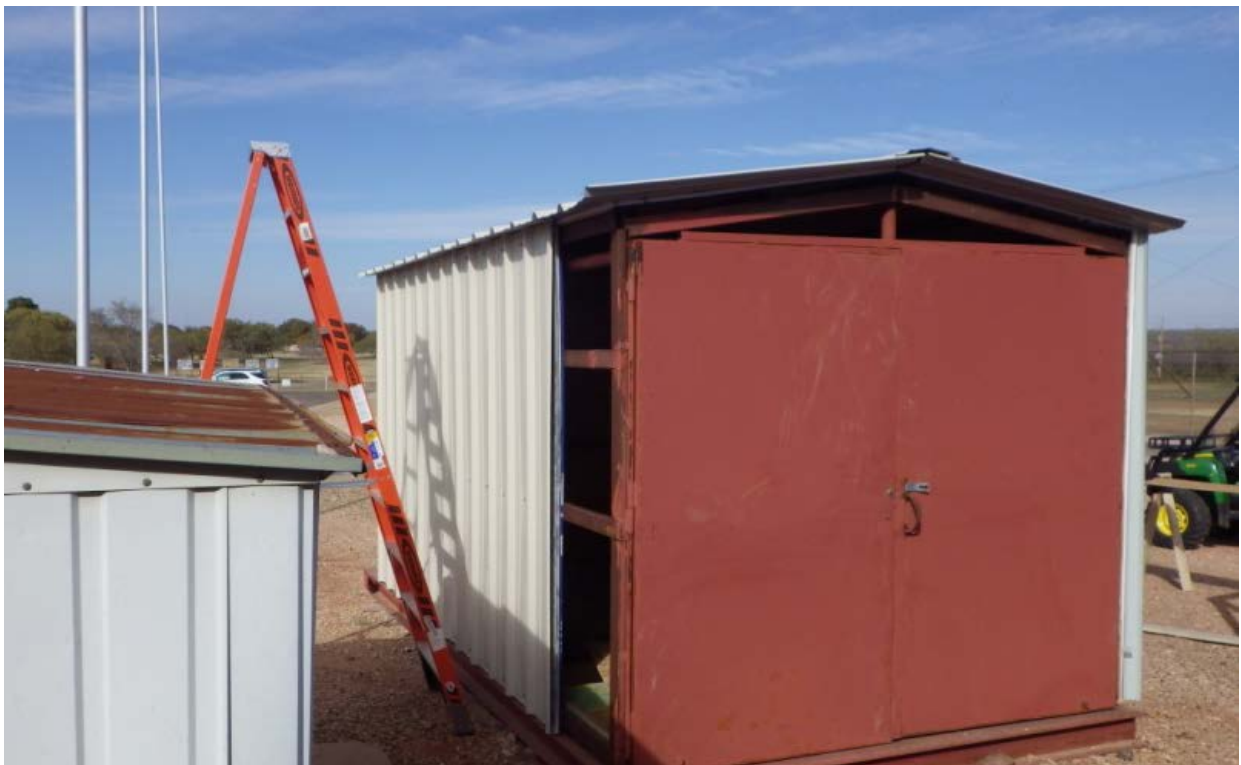
(Above) Nearly completed project.
